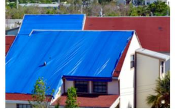
Roof waterproof cover
